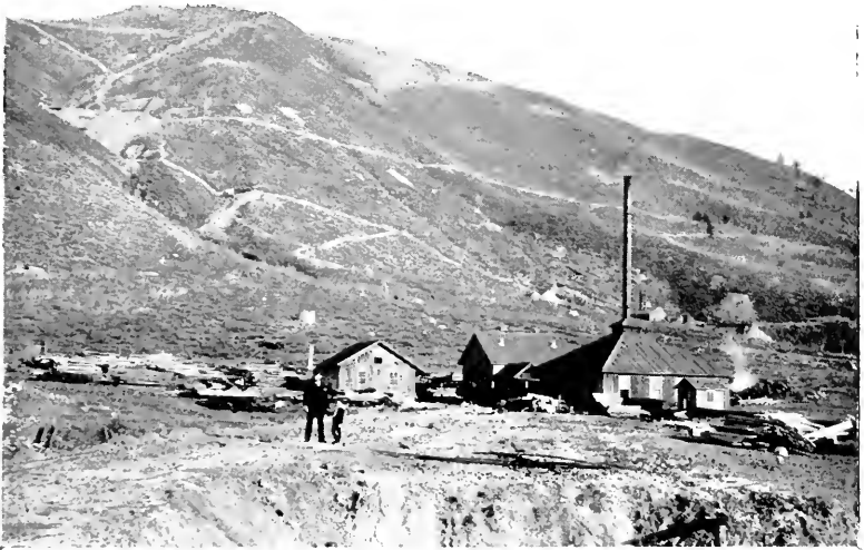
POWER-HOUSE, TIMBER-HOUSE AND BLACKSMITH SHOP, COWENHOVEN TUNNEL.
